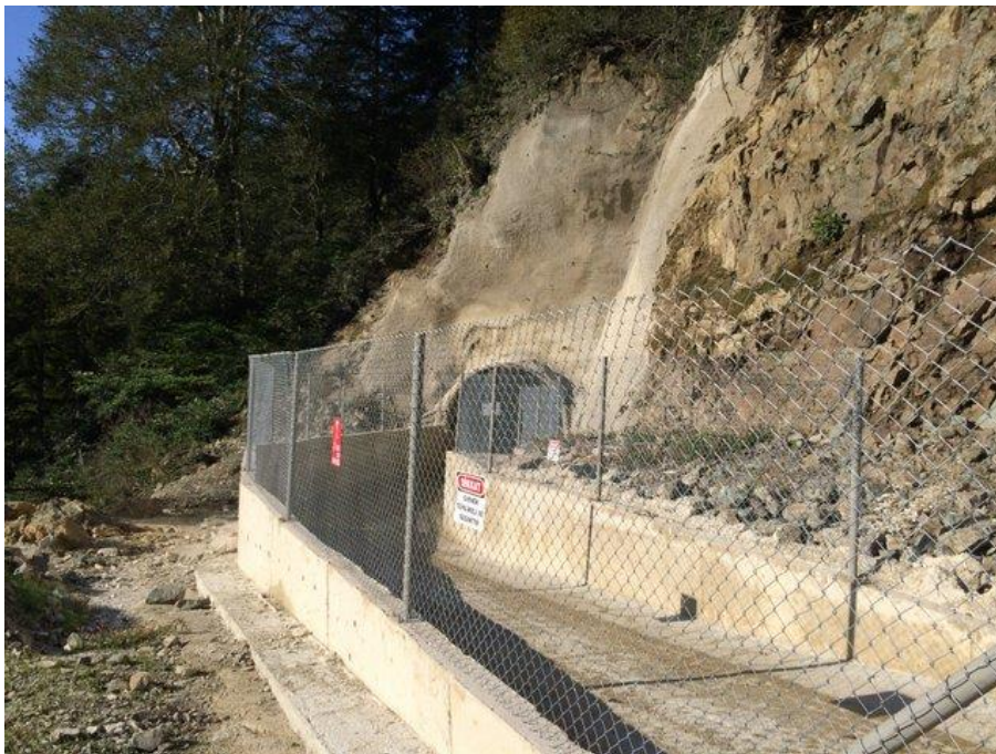
Figure 5.8 Slope Stability Precautions -Tuğra-II First Tunnel Portal
