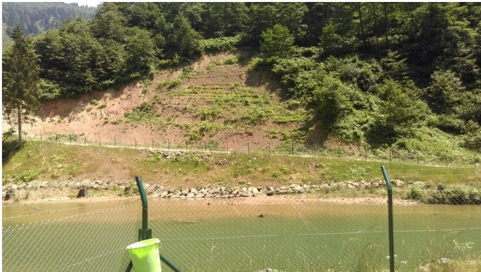
Figure 5.4 Environmental Safety Fence
