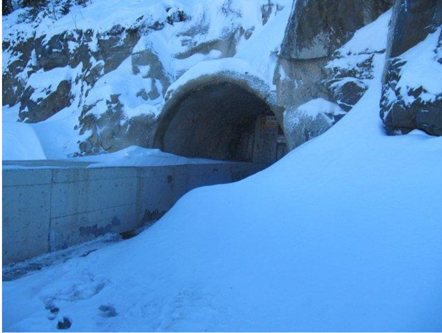
Figure 5.7 Slope Stability Precautions-Tuğra-I Tunnel Exit
