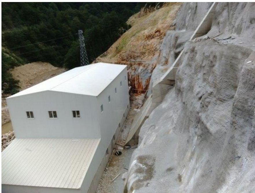
Figure 5.10 Slope Stability Precautions -Tuğra-II Powerhouse
