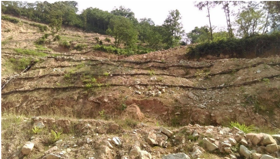
Figure 5.2 Terraces for Slopes
