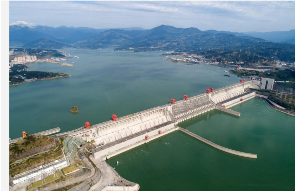
Figure 3.1 Three Gorges Dam 40
