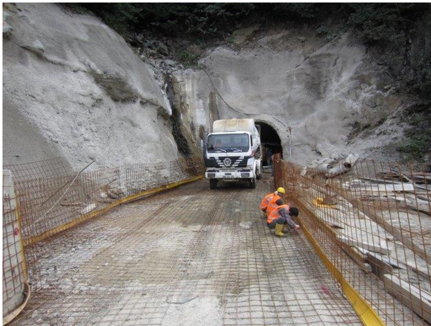
Figure 5.9 Slope Stability Precautions -Tuğra-II Second Tunnel Exit
