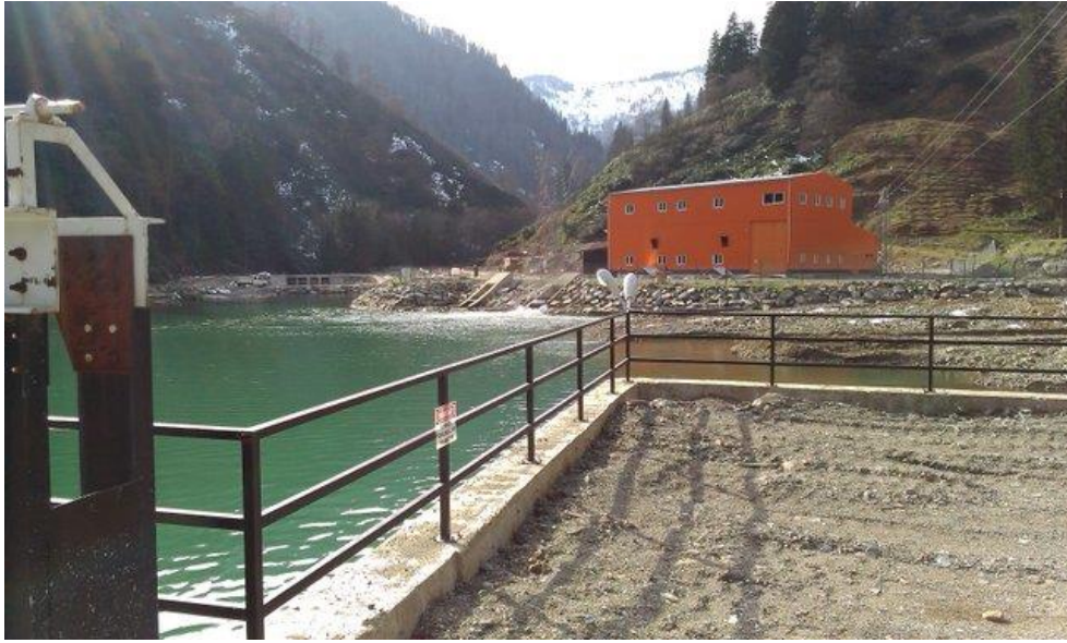
Figure 5.3 River Bed Reclamation
